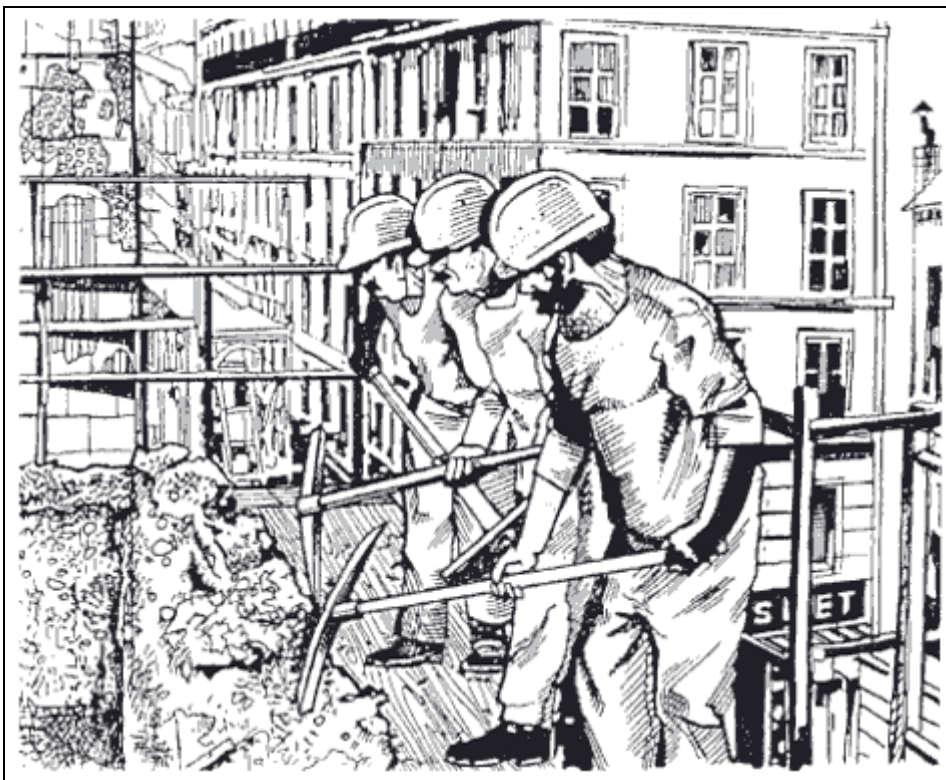
Figure 30. A scaffold platform from which demolition may be carried out safely
