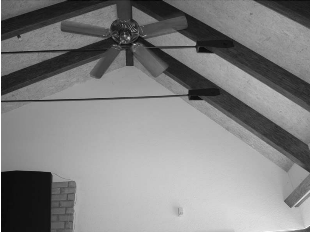
Figure 7.3 Exposed beam ceiling inside of 45° slope roof.
