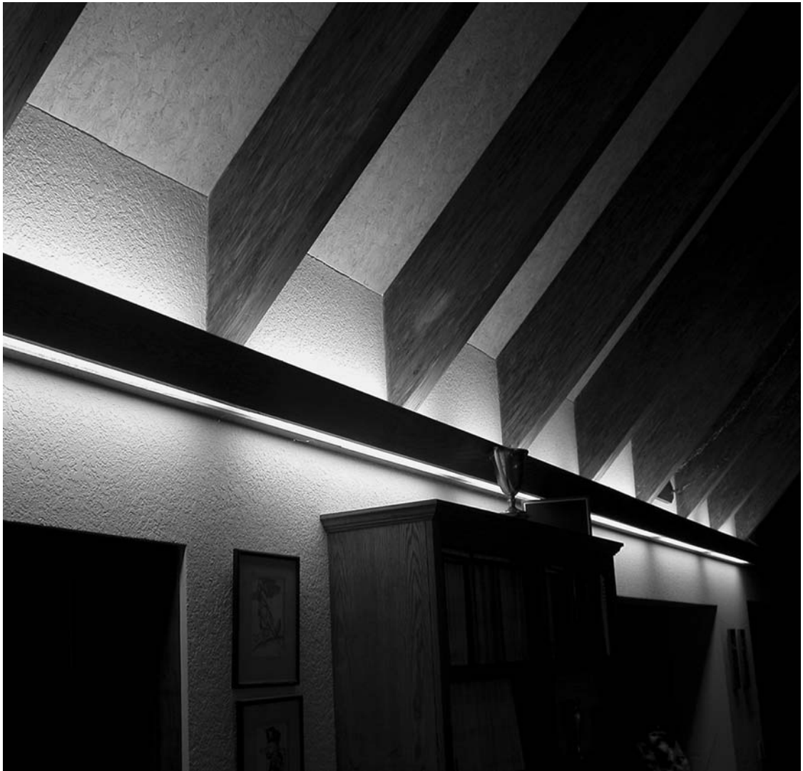
Figure 7.13 Photograph showing soffit lighting of ceiling rafters.
