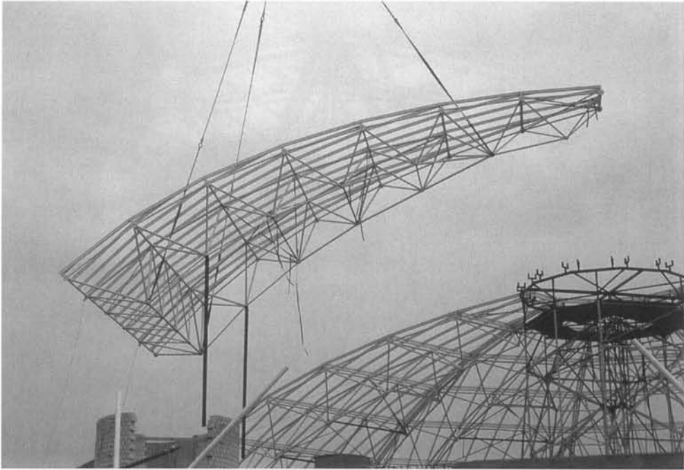
Fig. 8.21. A segment of the dome during hoisting
