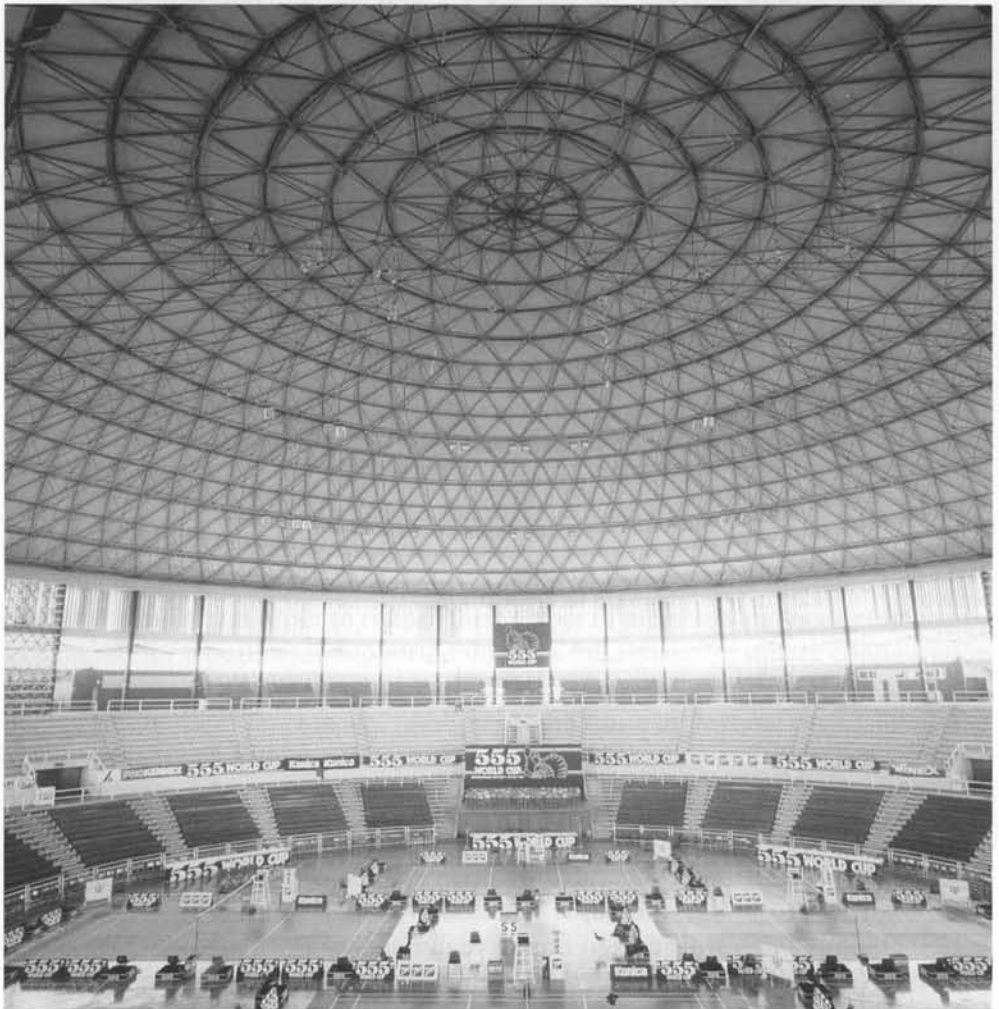
Fig. 8.19. The completed dome of the Negera National Indoor Stadium, Kuala Lumpur
