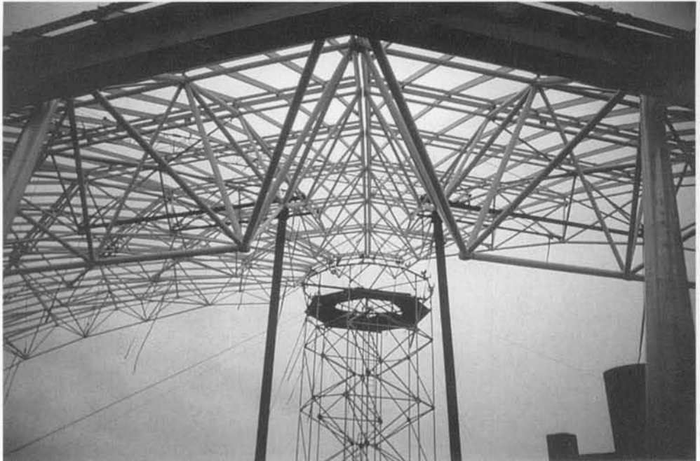
Fig. 8.22. The temporary space frame tower support
